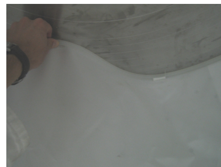
installation of the back PP hoop
